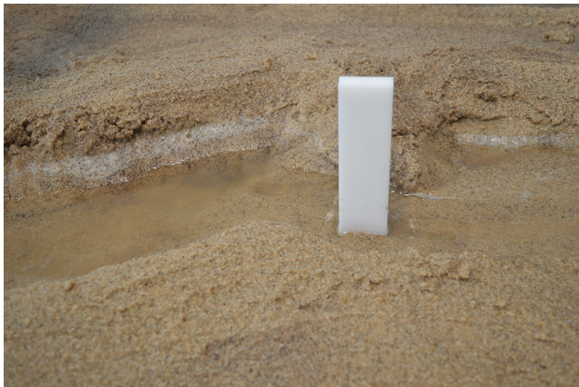
BRIDGE PIER SCOUR
